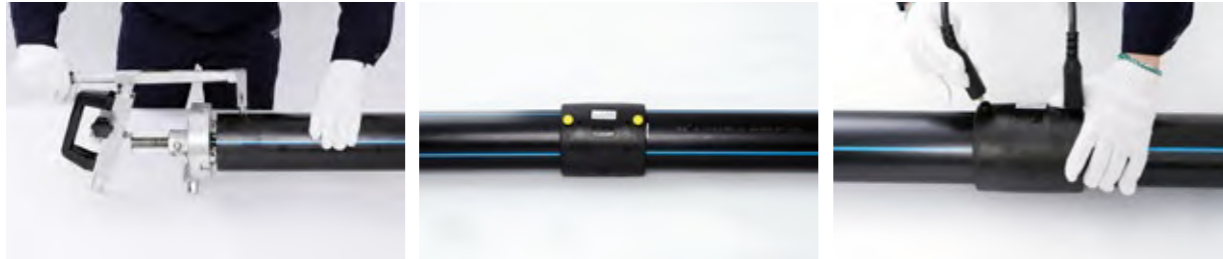
Cleaning &amp; peeling
